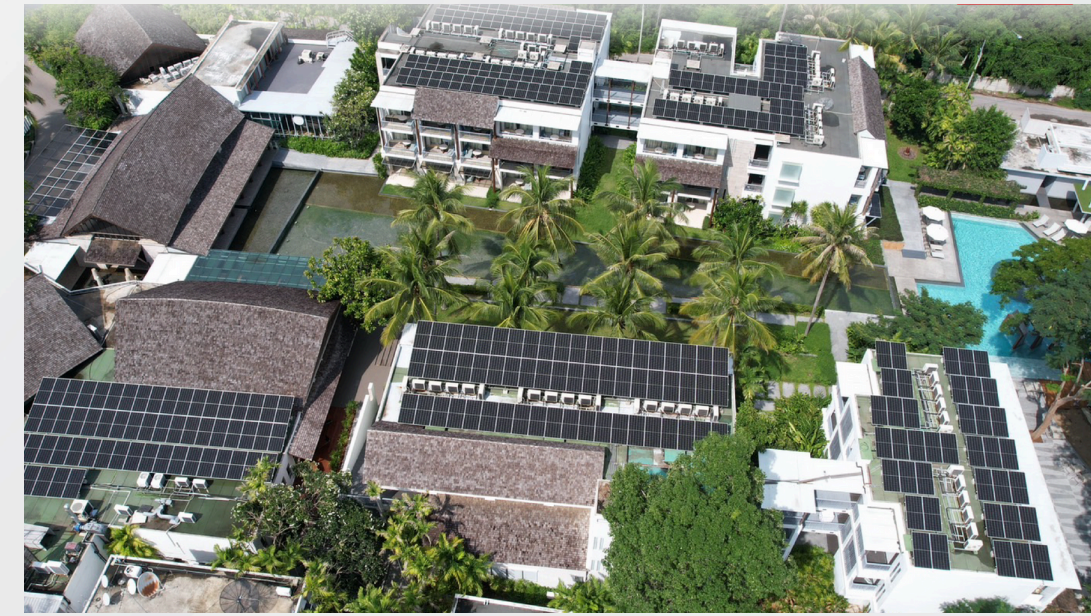
189.20 kWp Veranda Resort Huahin ,Cha-am
