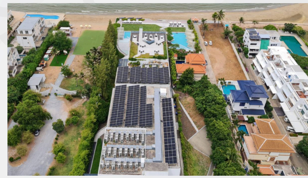
118.80 kWp Veranda Resort Pattaya
