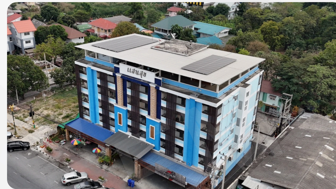
32.51 kWp Sansuk Apartment
