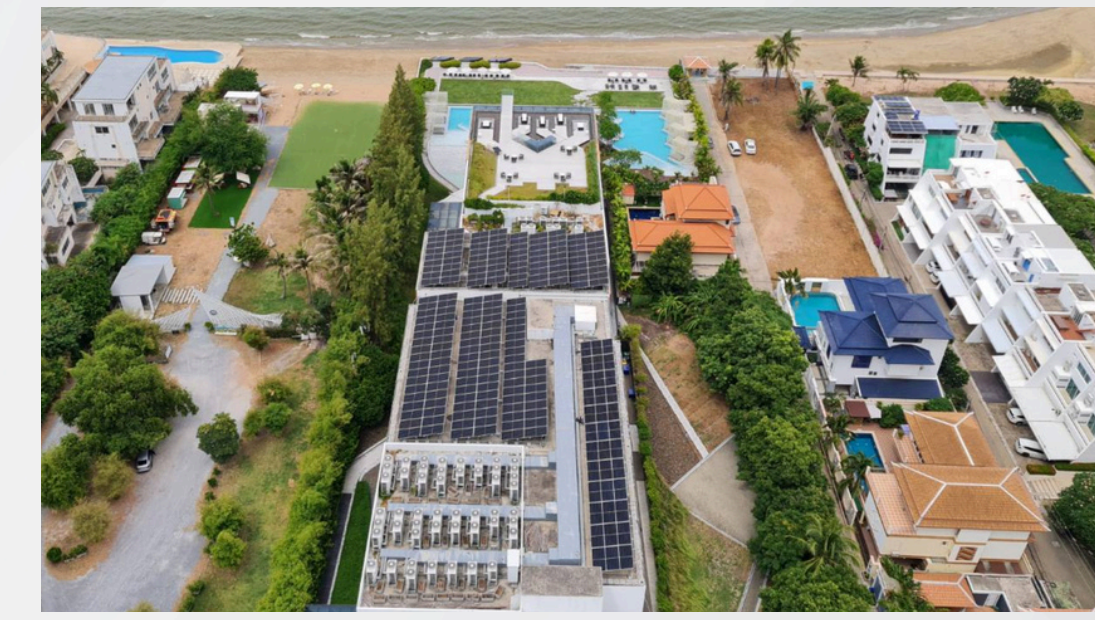
118.80 kWp Veranda Resort Pattaya
