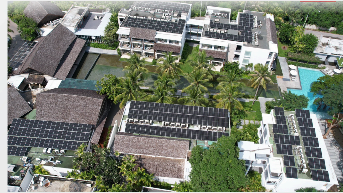
189.20 kWp Veranda Resort Huahin ,Cha-am
