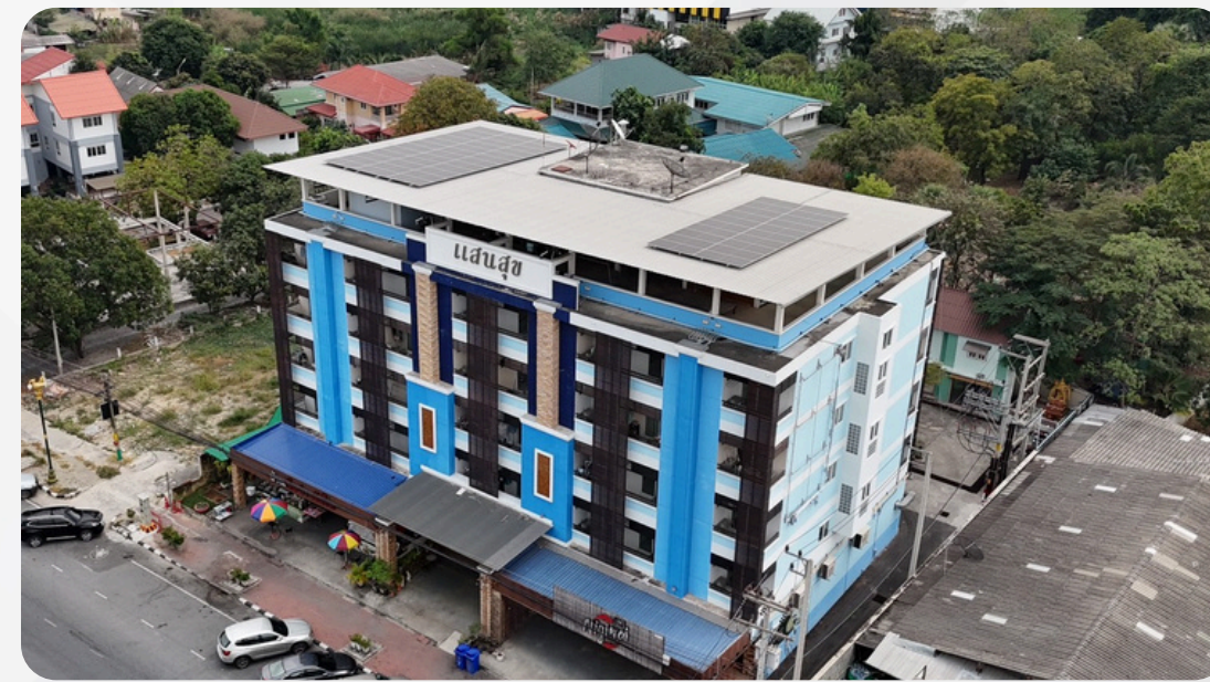
32.51 kWp Sansuk Apartment
